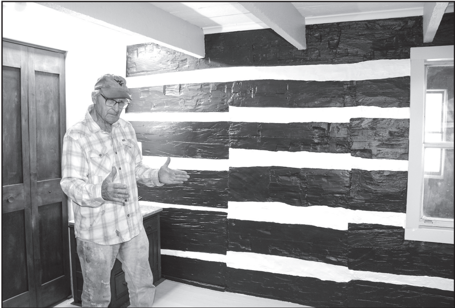
Charles Caldwell, Jr., describes the manner in which timbers were sawed. The original cabin featured a door in the mismatched area.
