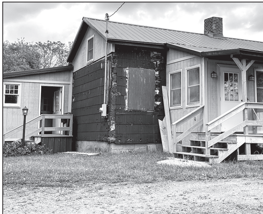
Asphalt siding of the 1950's hide the hand-hewn logs of the 1850's.
