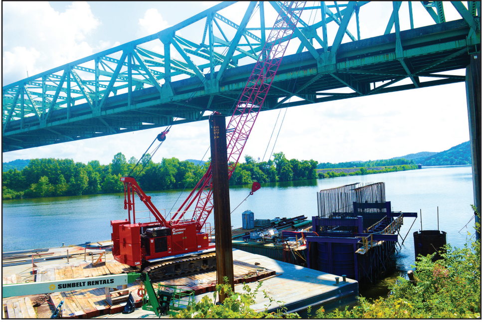
Pier construction at the western bank of the Kanawha River.
