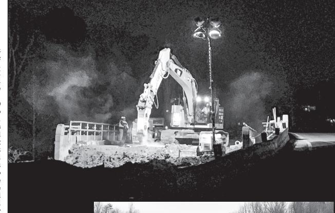
The above photo, taken January 11 by Ed Conner, captures the demolition of the old Bills Creek bridge over I-64. The demolition will allow I-64 to be widened to six lanes.
