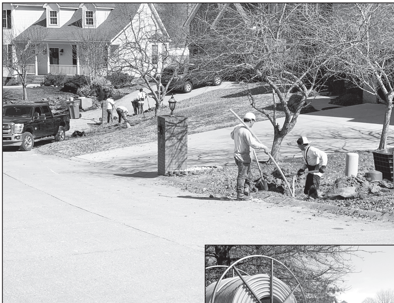
Right: The conduit pictured can carry over one hundred strands of optic fiber.
