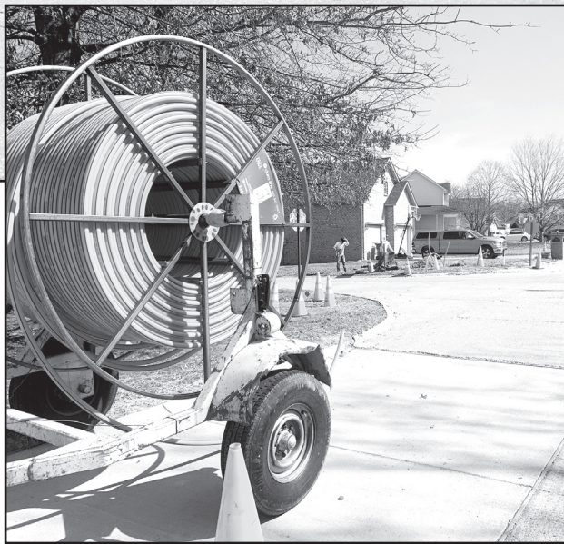
Right: The conduit pictured can carry over one hundred strands of optic fiber.
