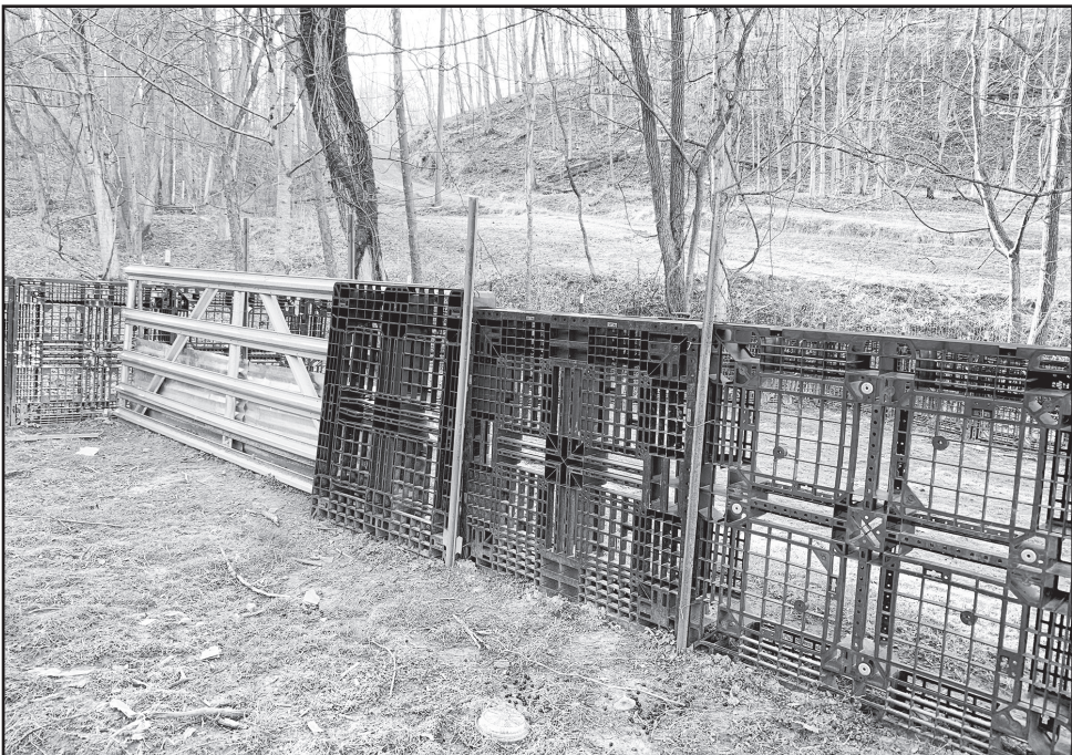
The pallets are joined with heavy duty plastic ties.
