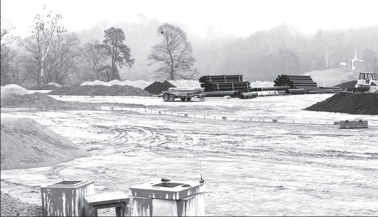
The plastic pipe is slated to provide drainage for the playing surfaces.
