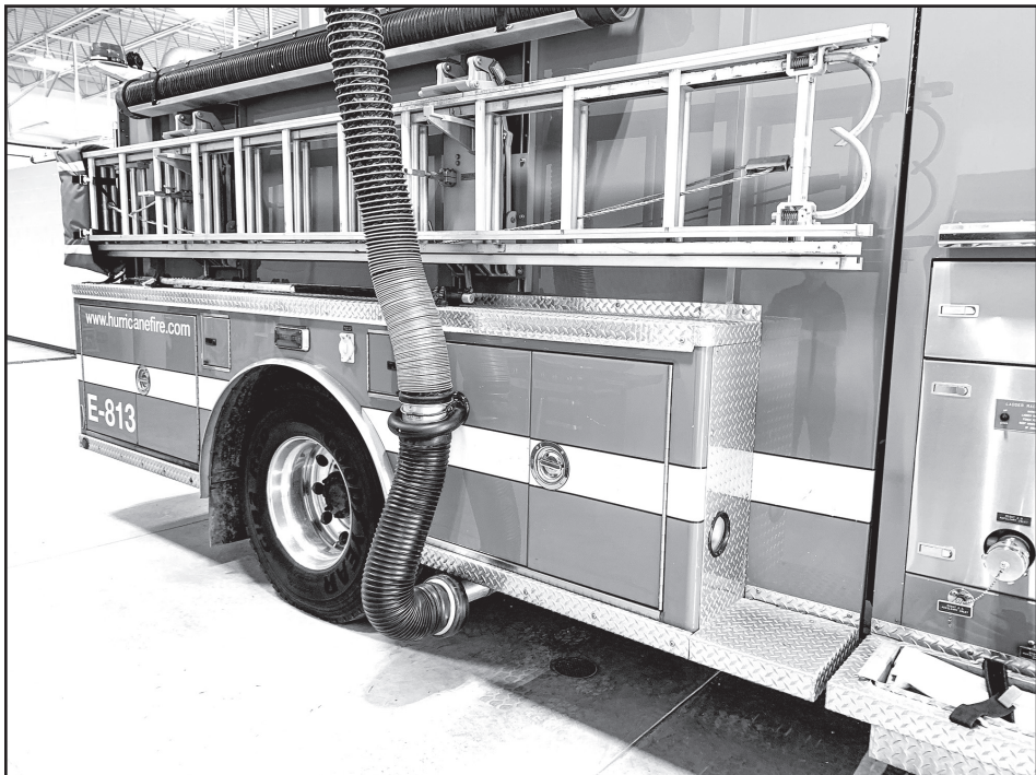
The station’s exhaust system activates when the ignition key is turned on.
