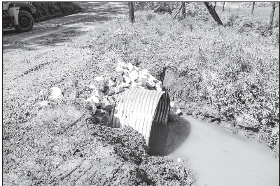
The new culvert is sized to put an end over-the-road water which has plagued motorists for many years.
