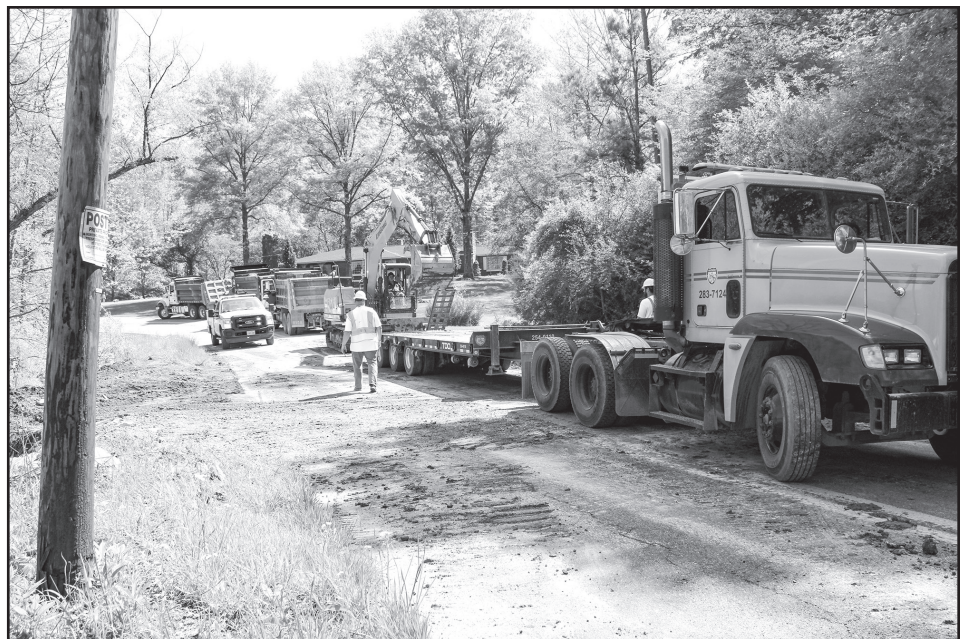
Hurricane Creek Road was shutdown Saturday morning (May 6) to allow workers to install a 48-inch culvert in place of a 30-inch culvert.
